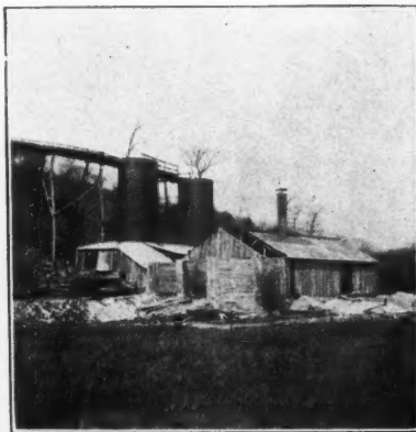
Kilns and Hydrating Plant Now Under Construction.
